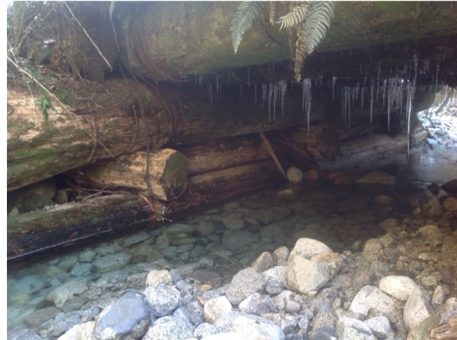
Left Bank Abutment when facing downstream
