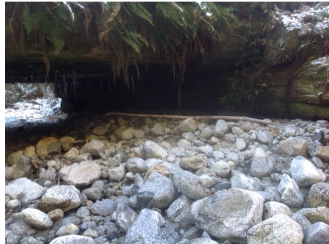
Right Bank Abutment when facing downstream
